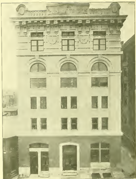
Masonic Temple of Fairmont, just completed by the Brady Construction & Engineering Company.
